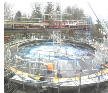
Water wrapping method
