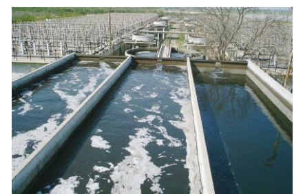
Agra Sewage Treatment Plant
