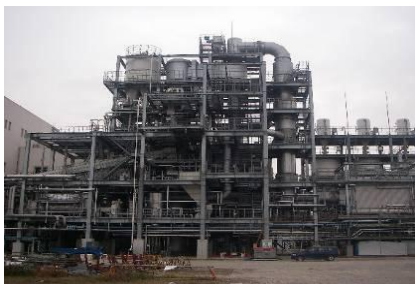
Sewage Sludge Incineration Plant ①City of Yokohama(Japan)②2007③200t/d
