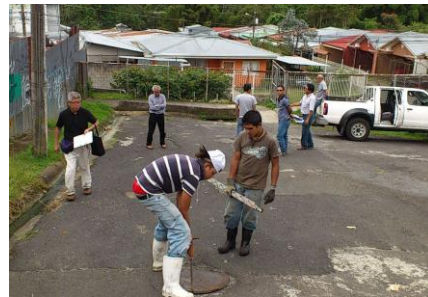
Investigation of existing MH in San Jose
