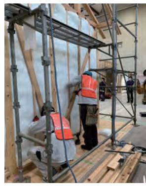
断熱施工の実技講習
